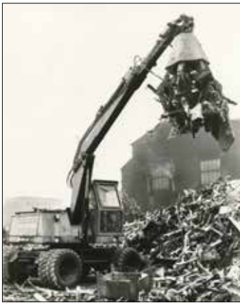
1967: SH 40 material handler in scrap operation
