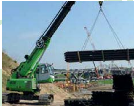
Civil engineering Tiefbau
