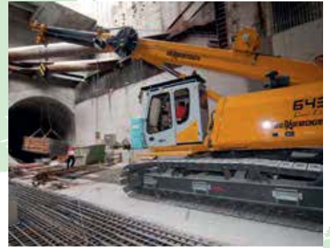
Tunnel construction Tunnelbau
